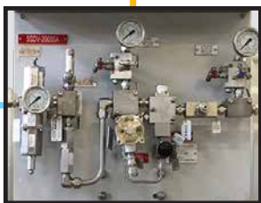
PNEUMATIC CONTROL PANEL
