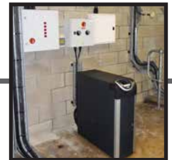
UNINTERRUPTIBLE POWER SUPPLIES
