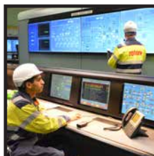
REMOTE CONTROL AND MONITORING
